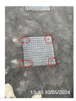
**Driveway** Inspection Lids Missing Screws Ground works contractor
