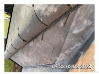
Low Level Roof Mortar Staines & Rubble Left On Roof Verge
