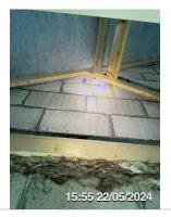
Internal Blockwork Gable Restraint Installed On A Cross Joint Nhbc 7.2.8 restraint straps must be installed behind a full block
