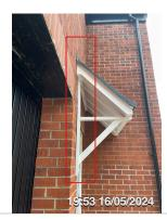
**Building** Brickwork Not Level & Out If Tolerance NHBC standards 9.1.2 8mm tolerance of a 25mm spacing block
