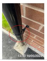
**Downpipes** Damaged Clip To Left Hand Side Downpipe Plumbing contractor
